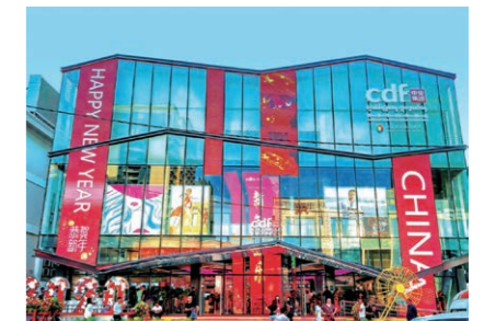
▲ cdf Sihanoukville International Airport Duty-Free Store
